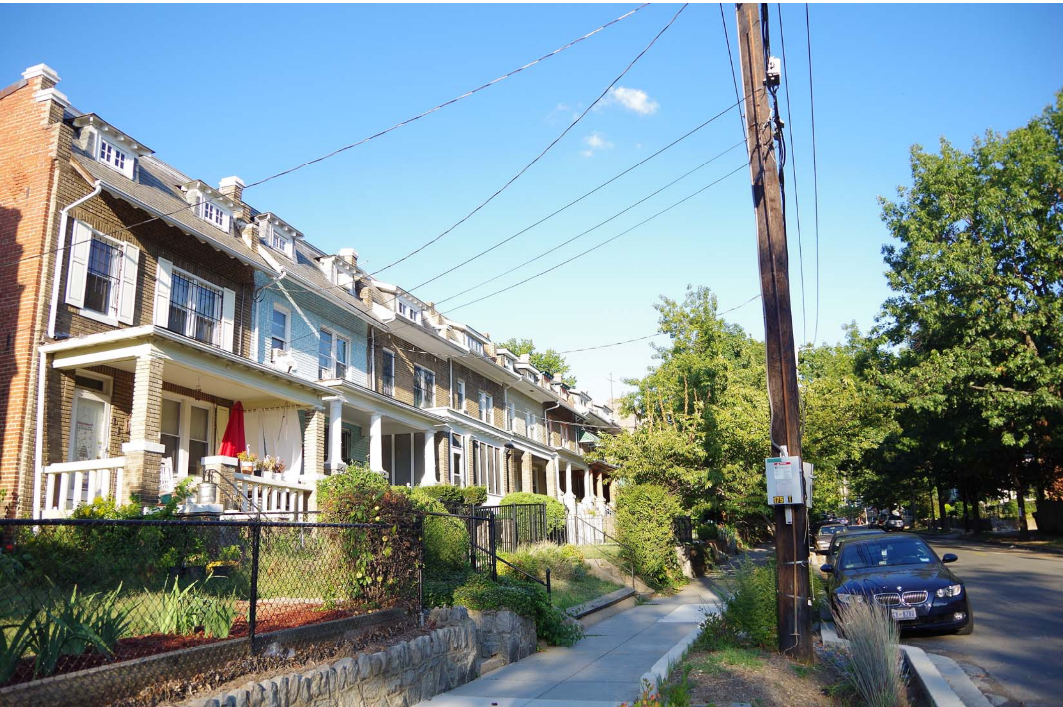
Front view of houses on 1100 block of Allison St NW
